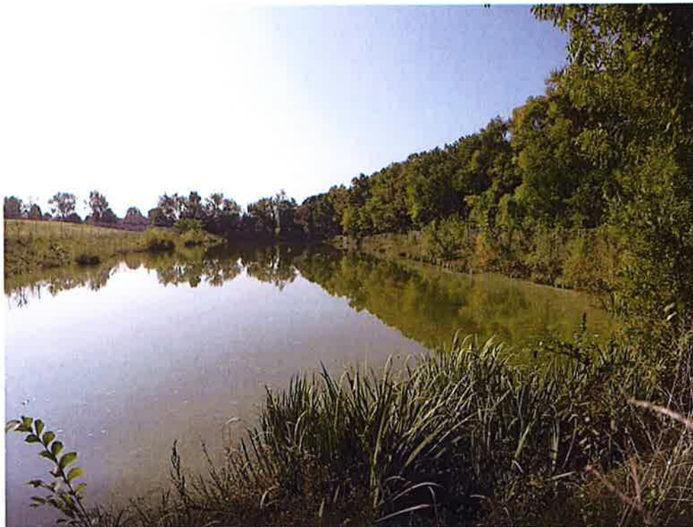
Photograph 6: Gumwood Road Retention Pond Water Level
