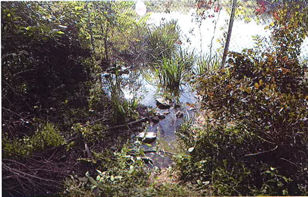
Photograph 5: Overflow into Gumwood Road Retention Pond
